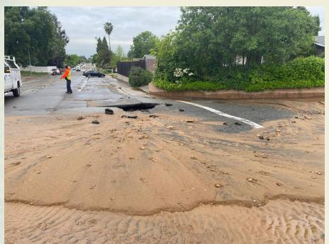
On the morning of April 24, 2024, instrumentation monitored by FOWD staff indicated a significant water pressure drop within the FOWD water system at approximately 5:50 AM. Field investigation by FOWD staff found that a 27-inch water transmission main located at the corner of Pershing Avenue and Chestnut Avenue was leaking and causing significant localized flooding and street damage.
